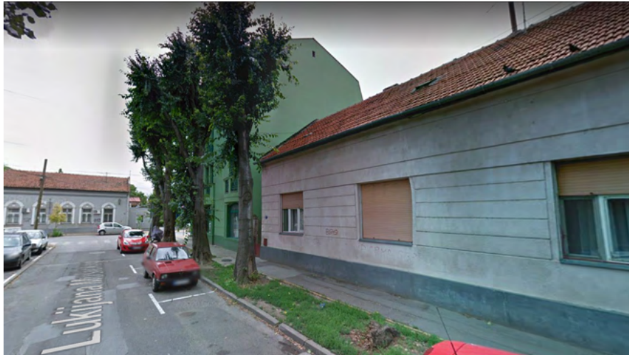
Neighbourhood:middle, Building: low, Source: Google maps
